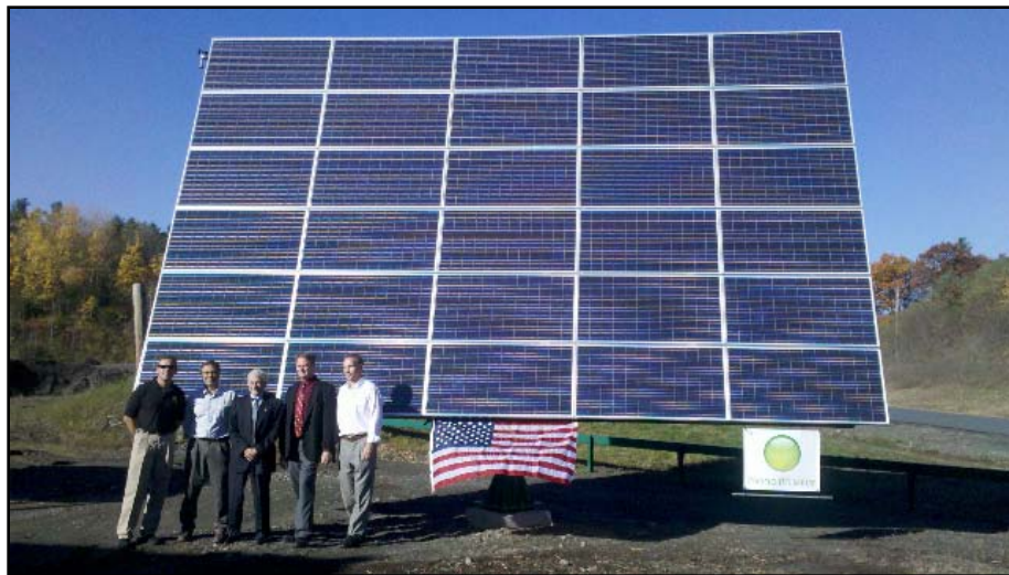
Solar Installation at the Town of Sand Lake, New York
